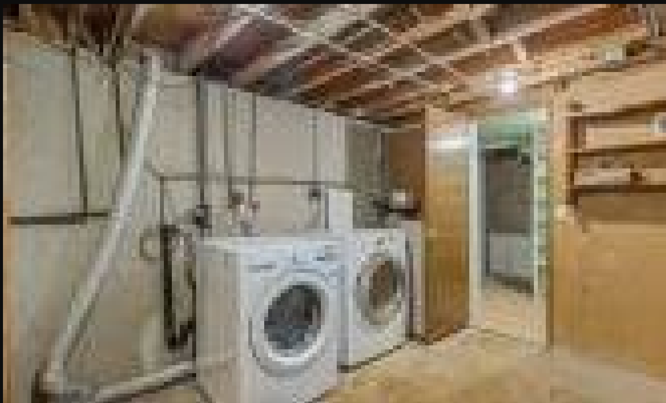
23 · Storage and utility area
